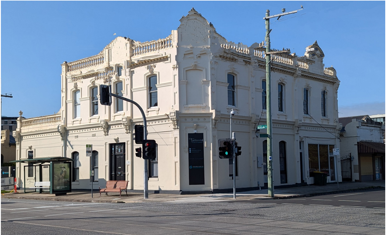
Prominently situated two-storeyed complex of 'Wybar Buildings' on the Balaclava Road/Kambrook Road corner. Erected 1887 by the Wybars as a bakery and commercial premises. May also have been a masonic lodge with a masonic symbol in the pediment. The verandah has been removed and shopfronts modified. Now Tailored Plastic Surgery. (Photo GEHS Collection 2024)
